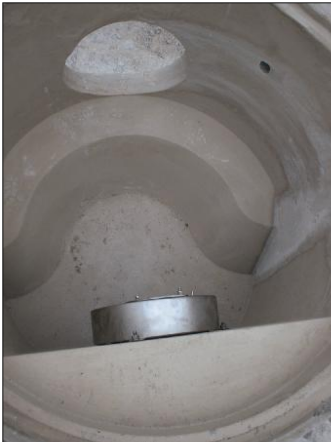
Figure 7. Hydro-Brake® vortex flow controls used to attenuate flows from ponds and infiltration devices
